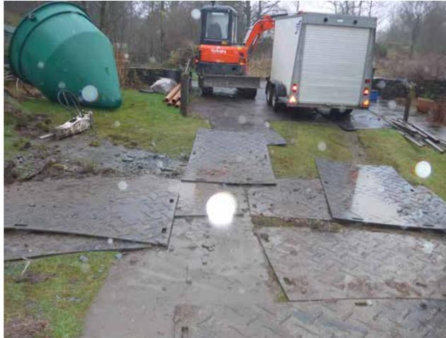
A specialist drainage firm was used to fix and clean the underground pipes, treating the insides of the pipes with a special coating. This was preferable to having pipes dug up and replaced. Removal of the old tank and installation of the new system took about 2 weeks. The new tank was installed on the site of
